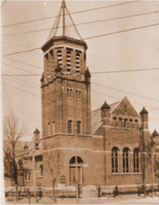
Murfreesboro Methodist Church (1888 building). No date, but this photograph was taken prior to the 1911 tornado which partially altered the church's exterior.
